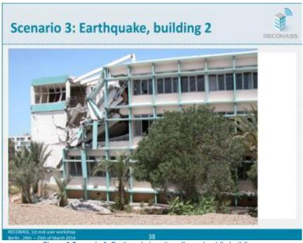
Figure 5-Scenario 3: Earthquake/ partly collapsed public buildings
